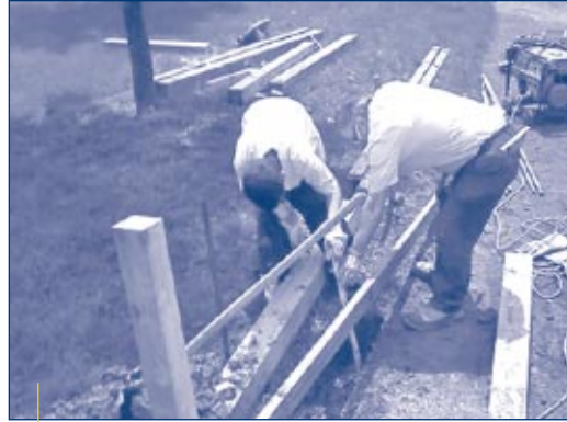
Work crew working in Upper Macungie Township
